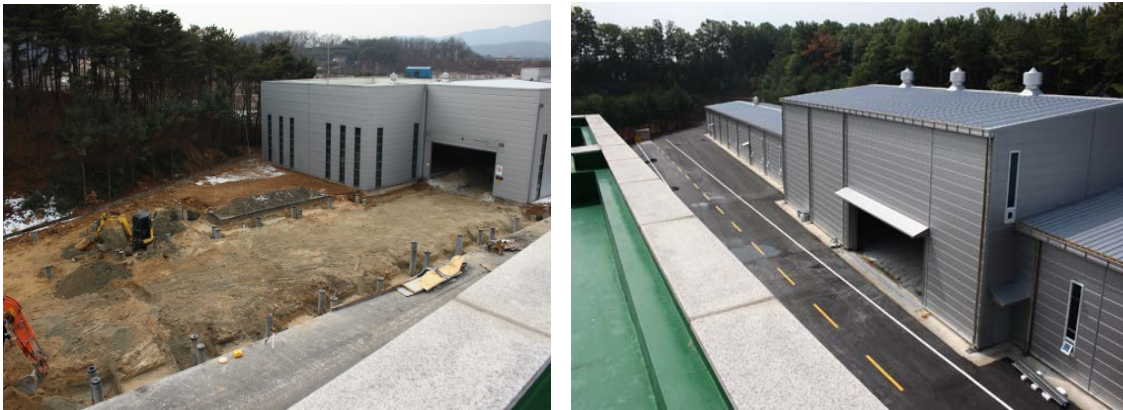
<Photo 1> New Crash Test Facility
