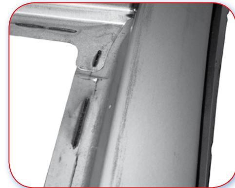
B.11.1 General example of laser welding applied close to flange edge.
