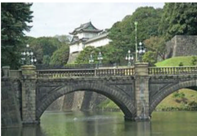
Nijubashi Bridge, A representative symbol of Tokyo
