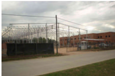
The Automobile Recycling Centre begins to take shape
