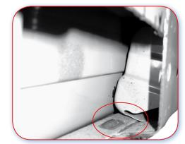
13.4.D Poor example. The sill cover panel runs to a bridging panel, not to the inner edge of the chassis/floor.
